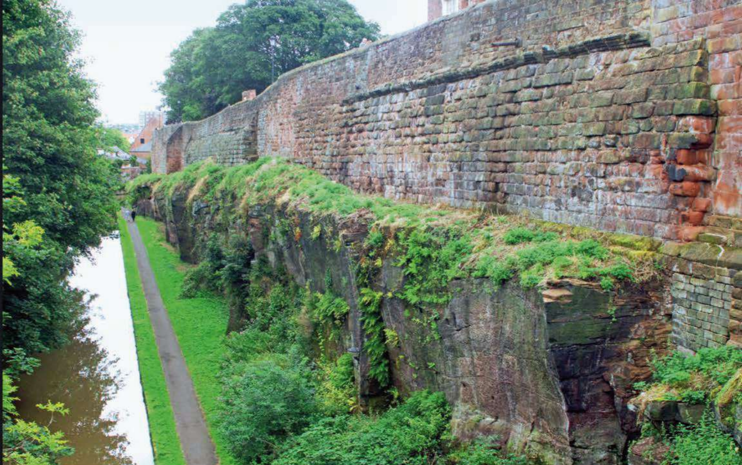
Chester city wall from Northgate to Phoenix Tower showing the cornice and repairs. Much of this section of wall dates back to Roman times.
